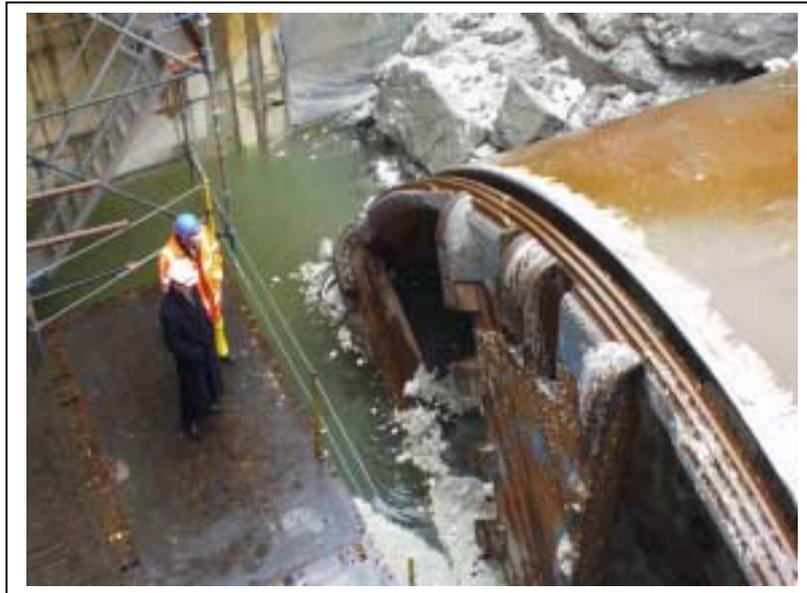
*Fig. 19: Mixschild for Westerscheldr / Netherlands / ( $\varnothing$  11,3 m) entering the reception shaft*
